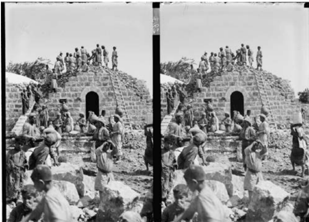
Figure 5. Stereograph of communal building practices in early twentieth-century Palestine. Photographer unknown, “Building Stone House in Village in Hill Country,” Matson Collection, Library of Congress, online at www.loc.gov/pictures/collection/matpc/item/2019694942/ (accessed 22 September 2020).
