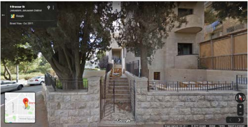
Figure 7. Screenshot of Google Street View for Said family house, now locatable at “10 Brenner Street,” seen here under construction, October 2011. Sokolov Square seen to the left, online at ( google.com ) bit.ly/311PhLJ (accessed 20 September 2020).
