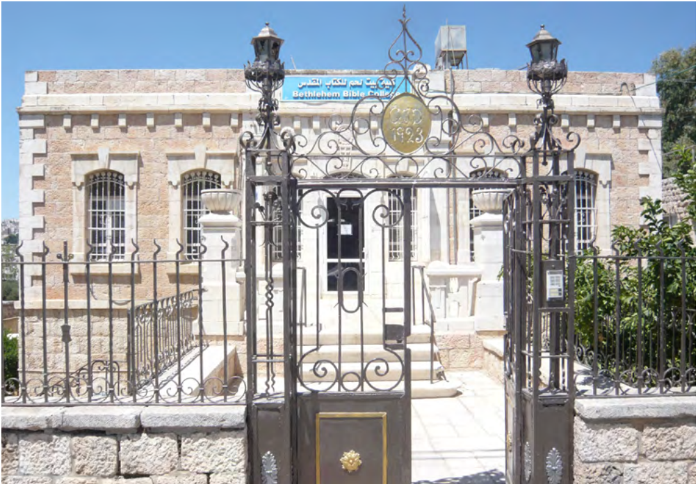
Figures 10 and 11. The houses built by Mikhail Dabdoub and Jubrail Dabdoub on Hebron Road, Bethlehem, in 1922 and 1923.
