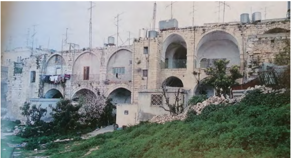
Figures 1 and 2. Hosh Dabdoub, as seen from street level (top) and from the valley to the rear (bottom); photo reproduced in Philippe Revault and Serge Santelli, “Typologie, Espaces et Composition des Maisons Traditionnelles,” in Maisons de Bethléem , ed. Philippe Revault, Serge Santelli and Catherine Weill-Rochant (Paris: Maisonneuve et Larose, 1997), 111.
