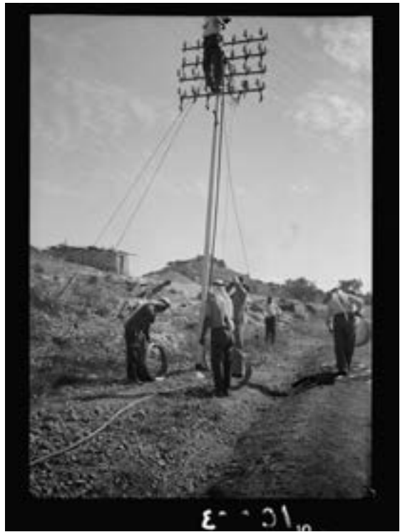
Figure 3. “Repairing telephone lines on Jaffa Road, 31 October 1938.” Matson Photograph Collection, Library of Congress, online at www.loc.gov/pictures/item/mpc2010004369/PP/ (accessed 29 May 2021).
