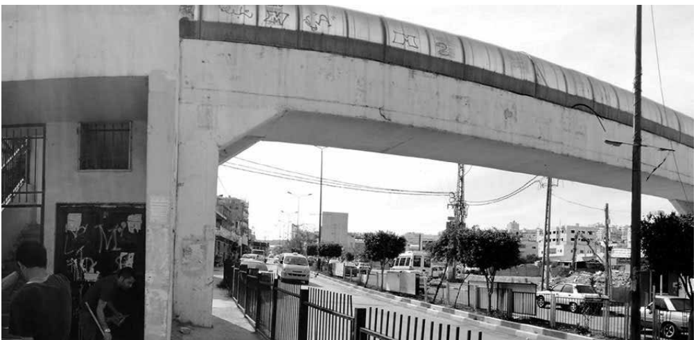
Figure 2. Dahaysha camp bridge. Photo courtesy of Campus in Camps, 2013.
