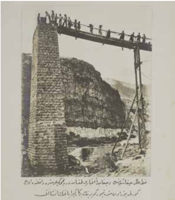
Figure 2. "The Haifa branch of the Exalted Line and construction of the stone column at the beginning of the three arched 110-meter-long railway bridge at the 94th kilometer of the Haifa branch" ( hat-ı ali Hayfa şubesinde ve Hayfa mebde itibarıyla doksan dördüncü kilometre dahilinde üç gözlü yüz on metre demir köprüünün bir kargir ayağının inşası ) shows workers on top of the temporary wooden bridge connecting the two main stone pillars of the bridge over the river in the Haifa branch of the Hijaz Railway. Source: Ömer M. Koç Collection.
